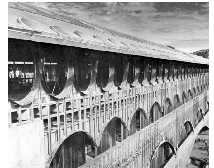
Marin County Civic Center, arches under construction
