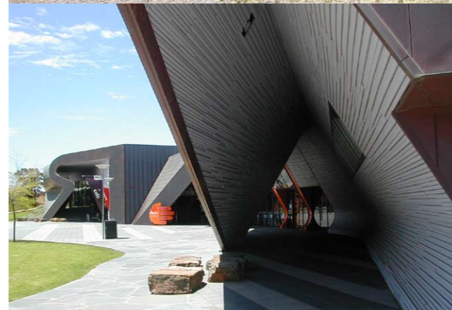
Marion Cultural Centre: 'MAR' letters on front elevation, arcade formed through the 'R' extrusion
