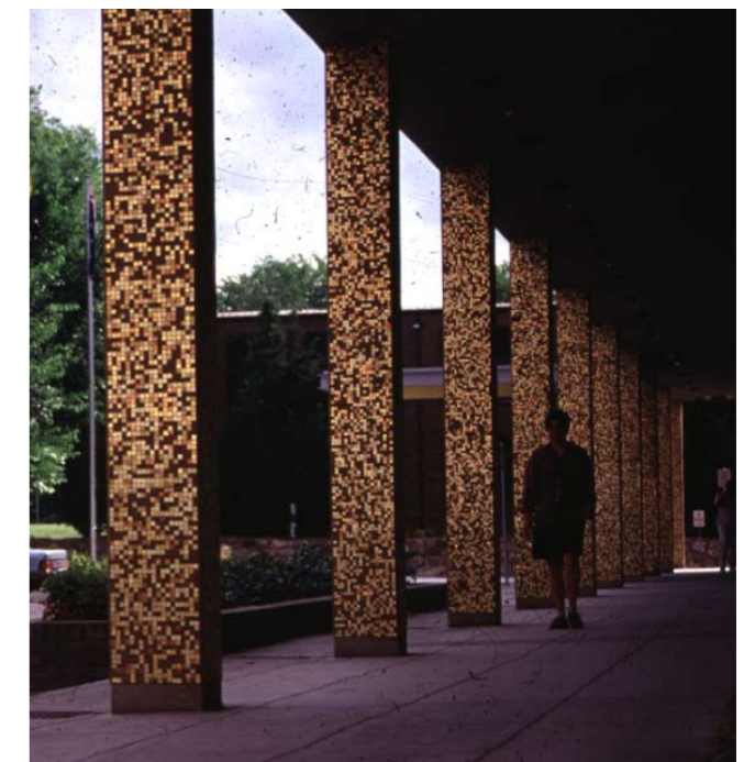
Canberra Civic Offices and Square, Yunken Freeman, 1961 uses gold mosaic tiling to the colonnade to distinguish itself from other modernist buildings in Canberra.
