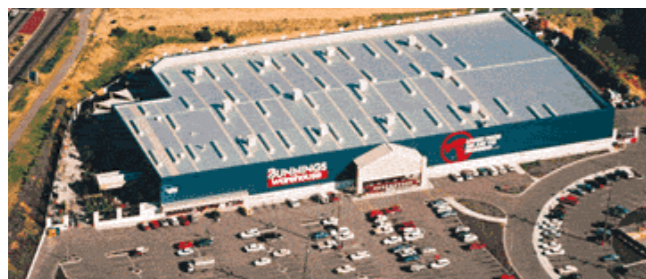
A typical Bunnings Warehouse from the air
