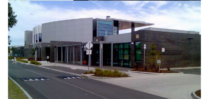
Carnegie Library, covered walkway from carpark to entry; rear elevation facing residential area
