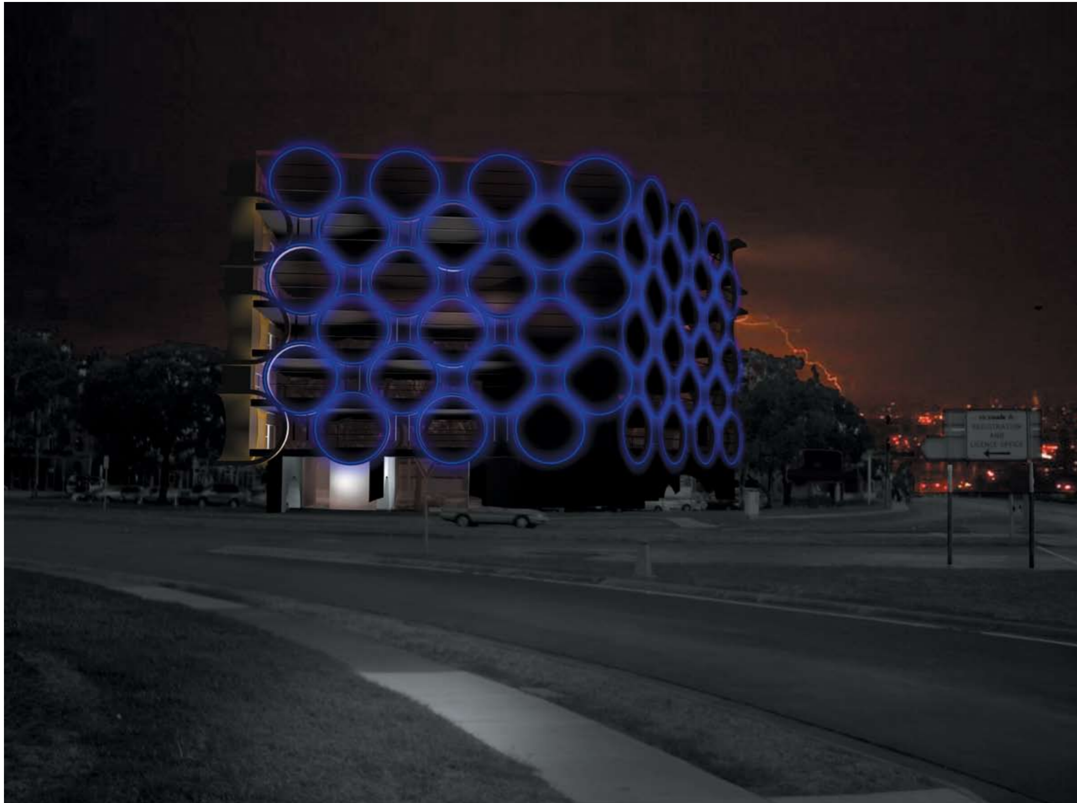
Night view from south-east, the common approach to site for motorists and train users.
