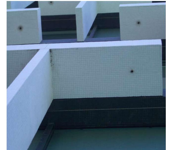
Detail of Council House 'Ts, cladding in white mosaic tiles
